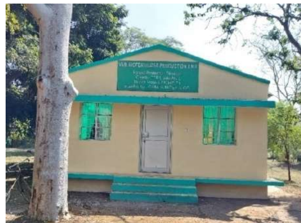
VAM production unit at ICFRE-TFRI, Jabalpur
