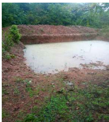
Fig 2 : Soil and moisture conservation works in Karnataka from the CAMPA funds
