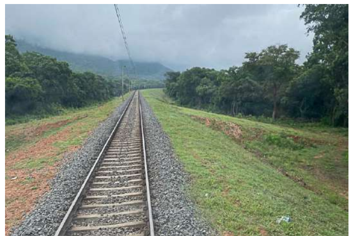
An example of a ramp built for aiding elephant movement across a railway line near Coimbatore, Tamil Nadu, India
