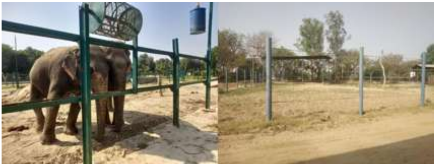
Enclosure barrier-I section girders (left) and High tensile wires (right).
