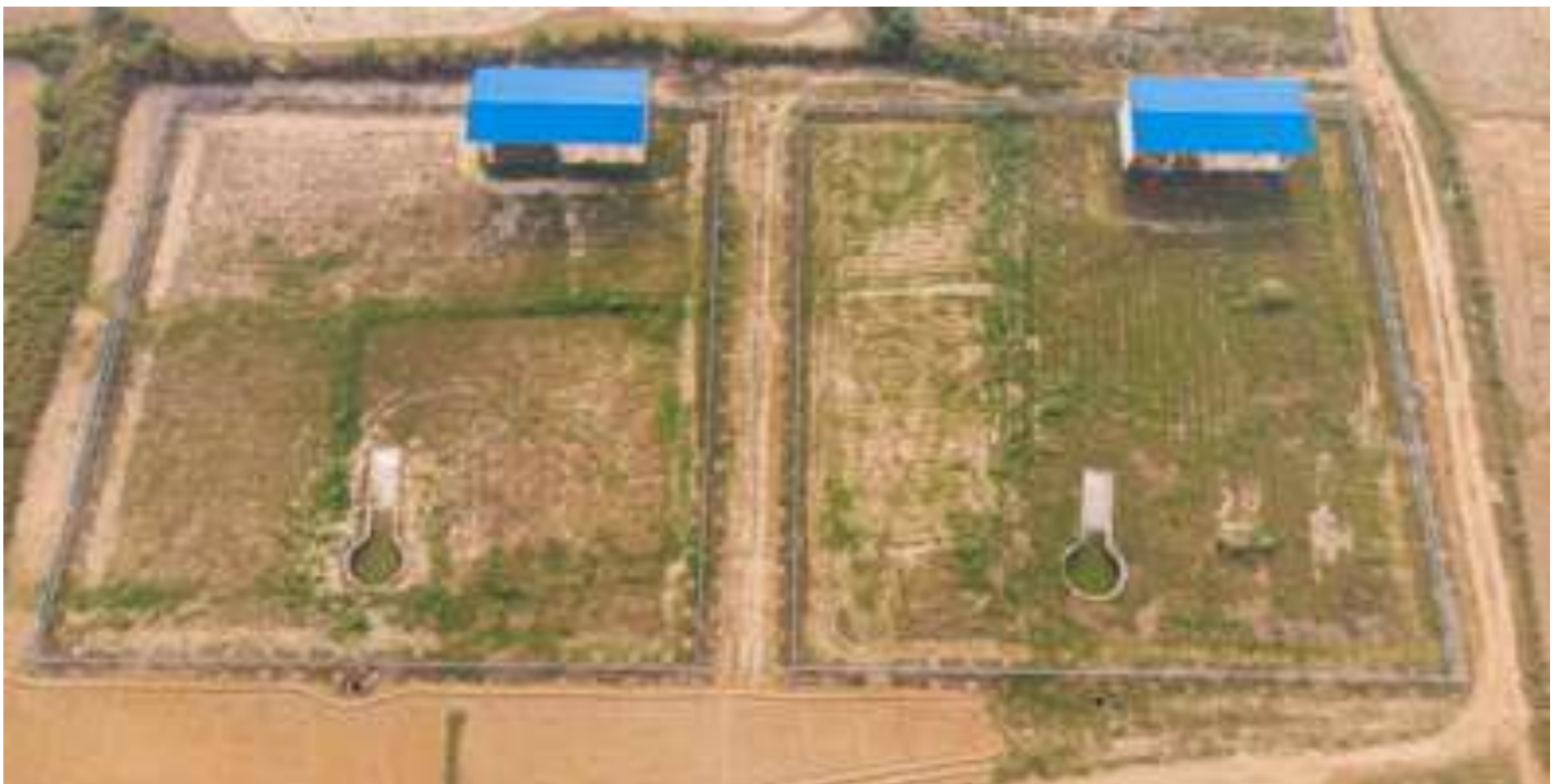
Overview of the enclosures.
