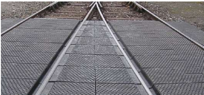
Figure 1. A level crossing with a rubberized surface that can be replicated on level crossings for wildlife.
