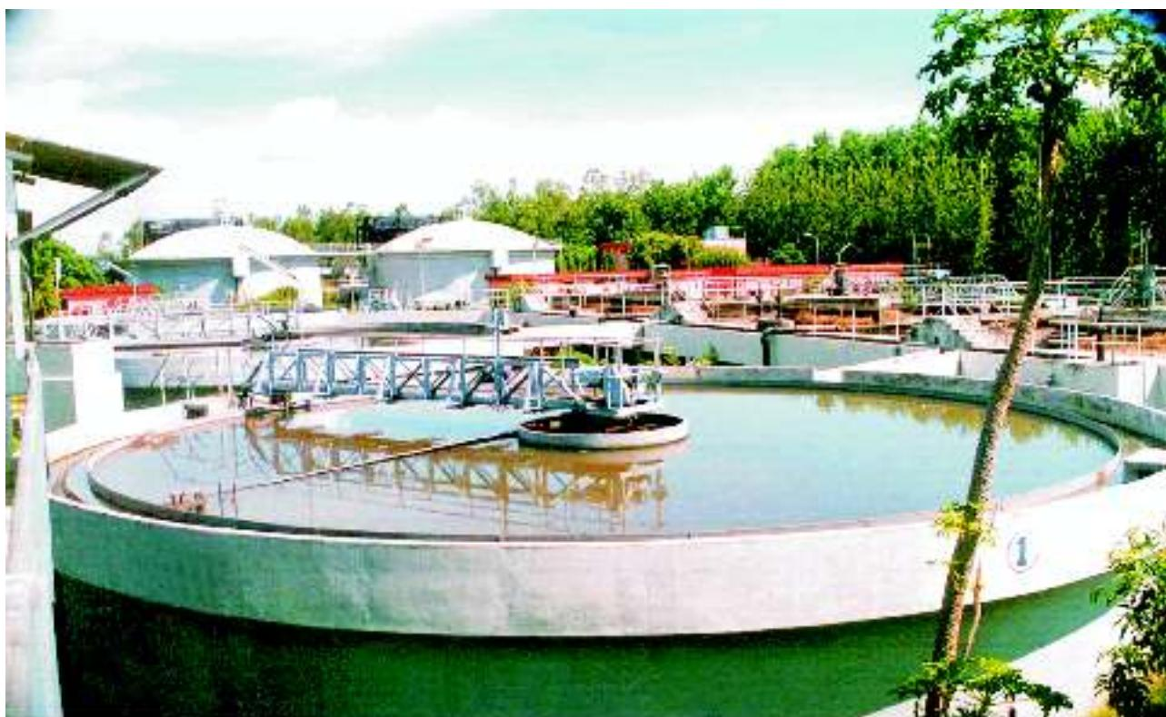
Fig-47. A view of Sewage Treatment Plant (Primary Clarifier) in Hardwar
