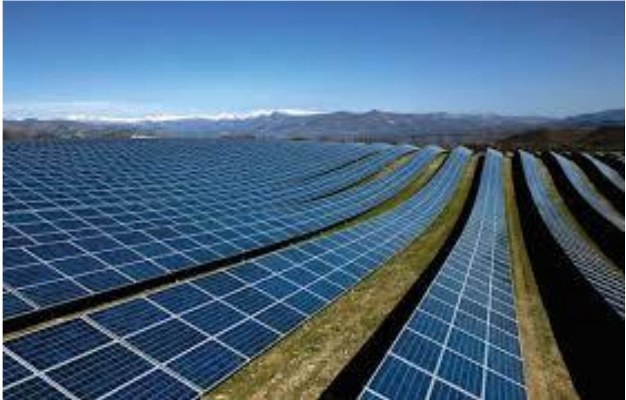
Figure 6.3: Rewa solar power project
