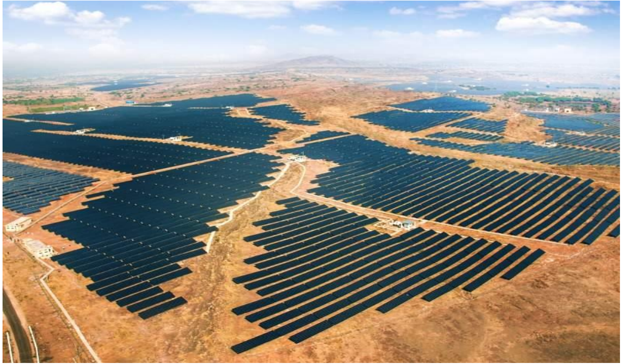
Figure 6.2: Bhadla Solar Park
