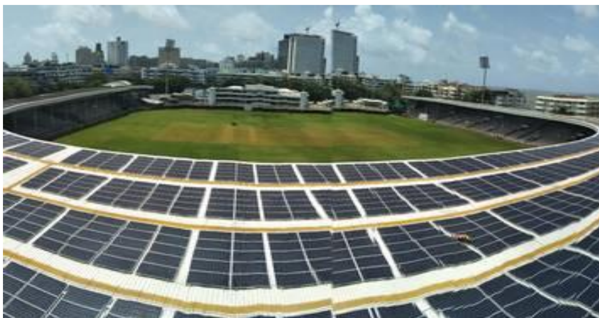
Figure 6.1: Solar rooftop of Brabourne Stadium, Mumbai
