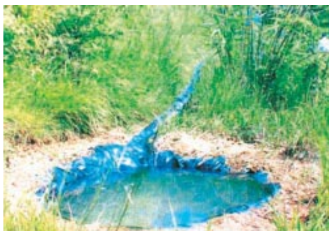
Fig 69. A poly-pond collecting water through a polythene lined minor canal for use in silvi-pasture development in Dugar Gad watershed in Garhwal
