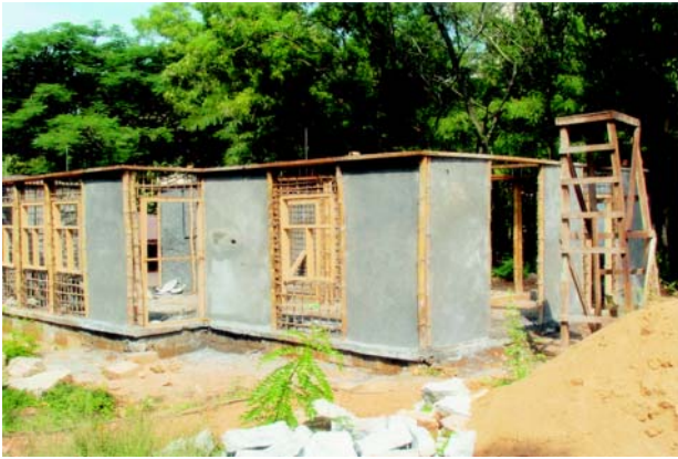
Fig 62. Two storey bamboo house construction
