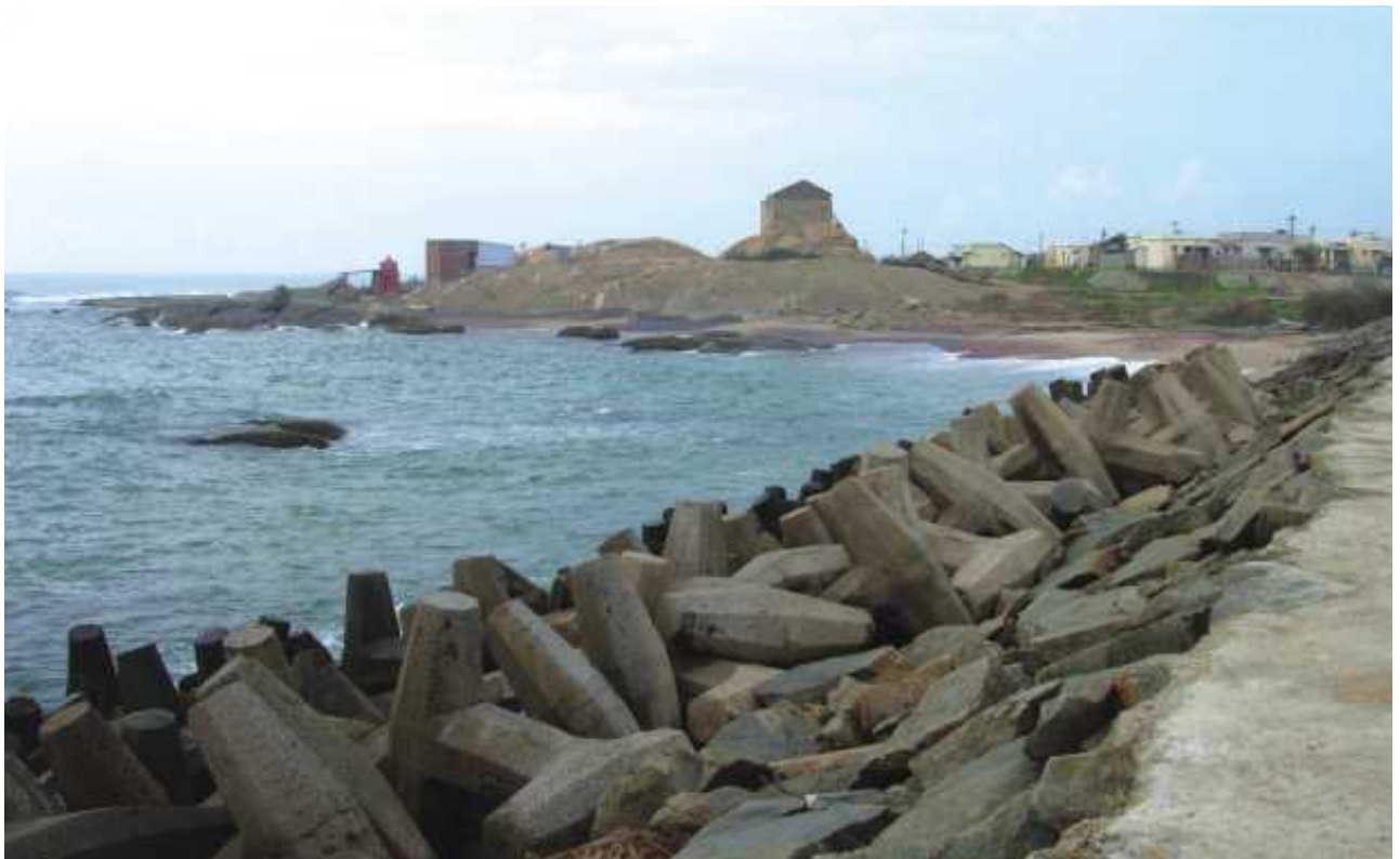
Fig.33 Prevention of coastal erosion at Kanya Kumari
