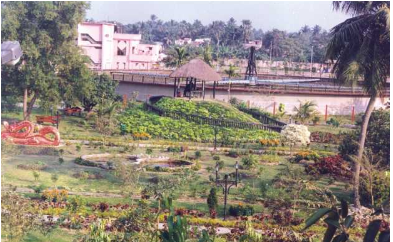
Fig.45 Sewage treatment plant with attractive surroundings at Chandan Nagar, West Bengal
