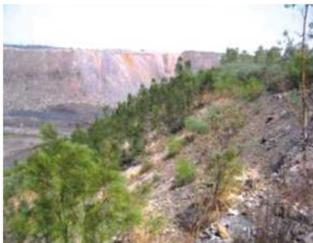
Fig.69 Slope stabilization in MCL
