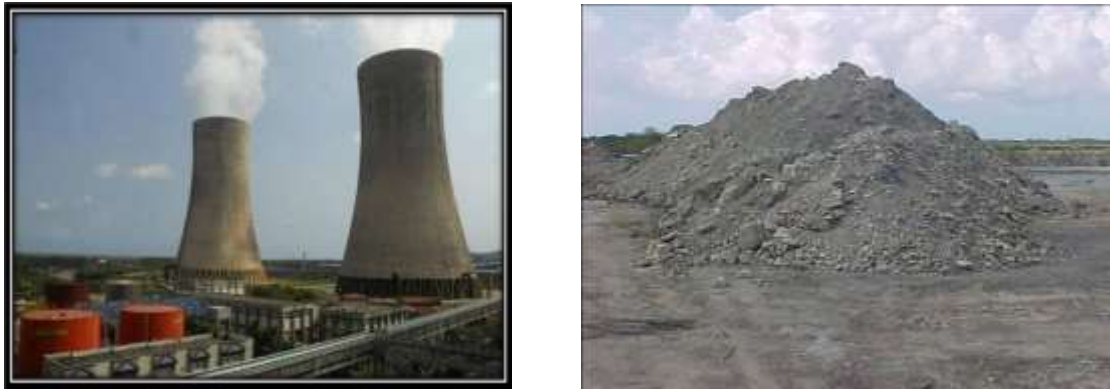
Figure 1. Shows thermal power plants producing fly-ash as a waste material
