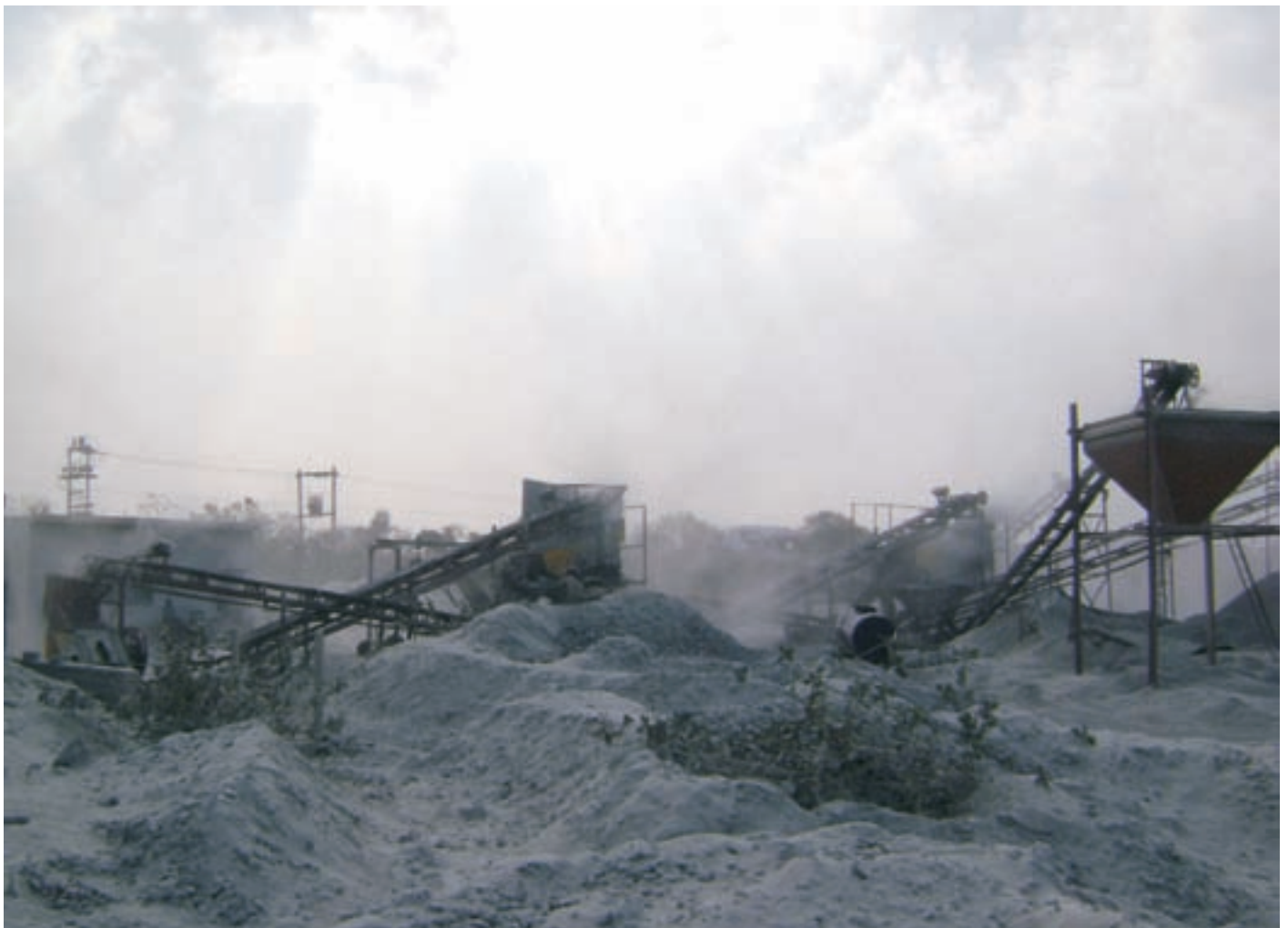
Stone crushing unit needs dust control systems to minimize air pollution
