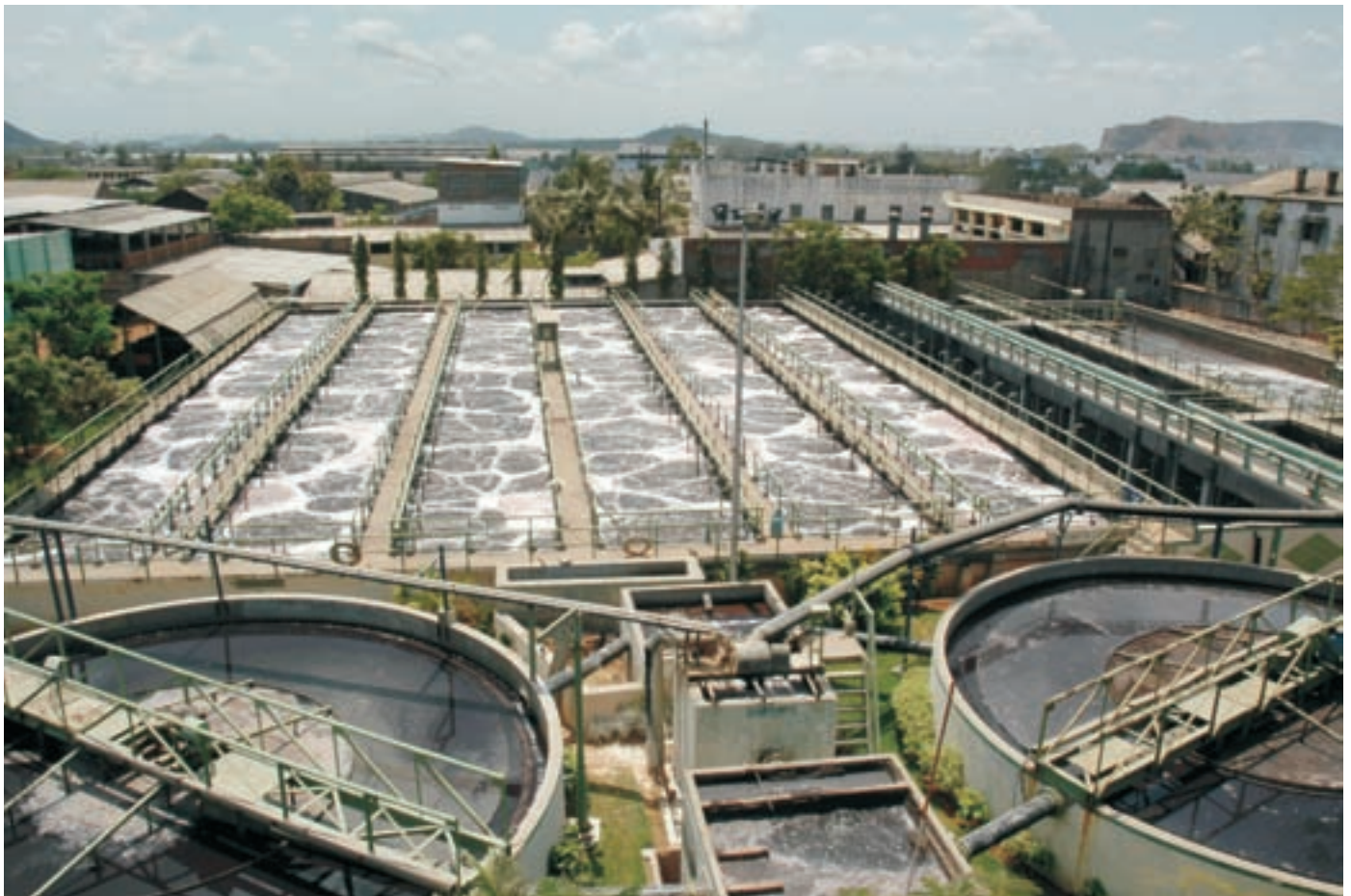
A common effluent treatment plant at Chennai
