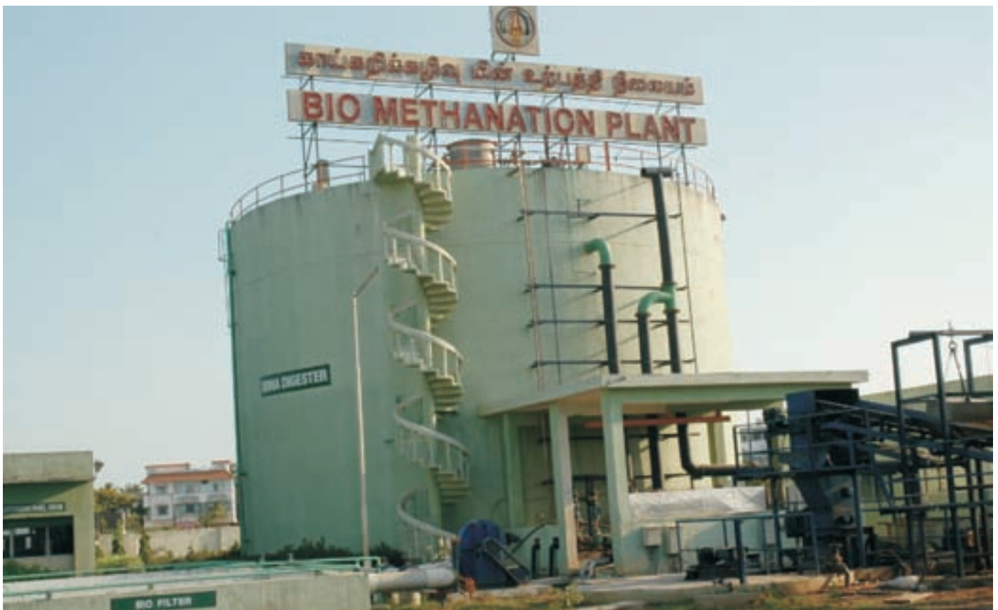
Bio Methanation Plant at Chennai
