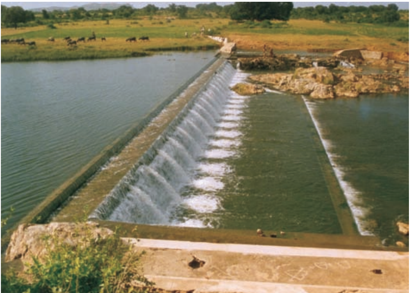
Check dam in Bundelkhand : Small is sustainable
