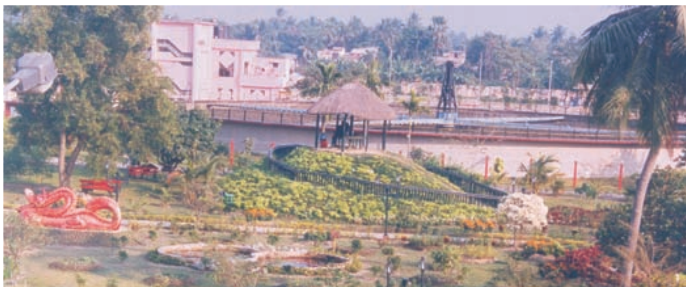
Sewage Treatment Plant with attractive surroundings at Chandan Nagar in West Bengal
