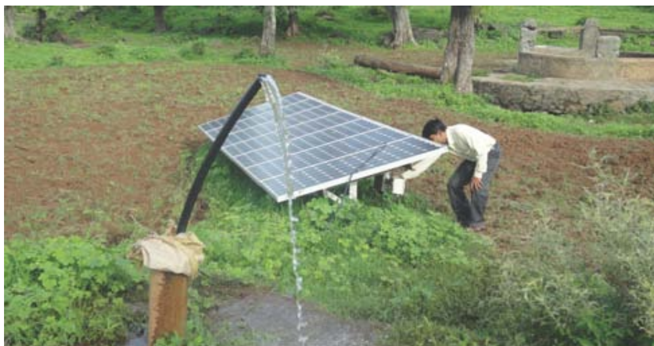
Water lifting by solar photovoltaic system, Kakshala, Dang district, Gujarat.
