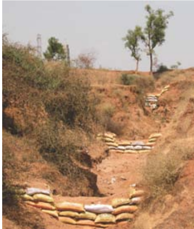
Boribandh treatment for ravine reclamation, Dunggripura, Savli block, Baroda district, Gujarat
