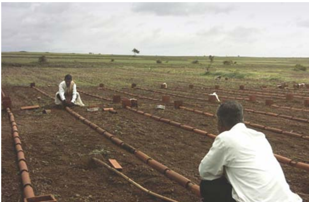
Innovative micro irrigation system in the villages of Jath block, Sangli district Maharashtra.
