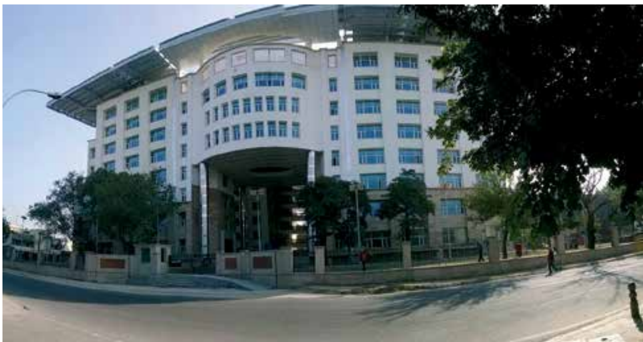
Fig-62. New Office Building of the Ministry at Jorbagh Road, New Delhi
