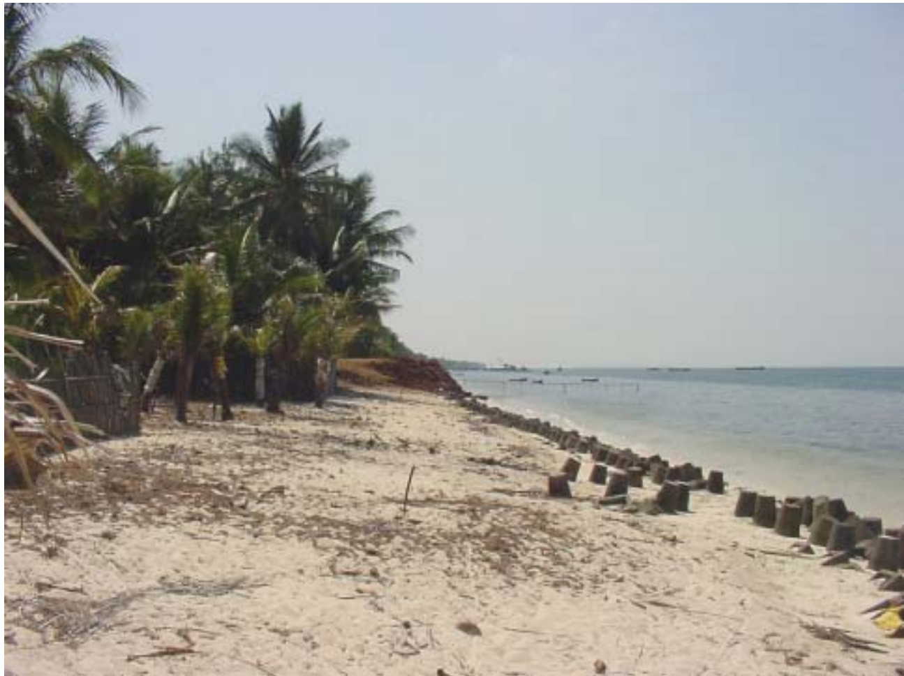
Fig-26. Protection structure to prevent coastal erosion
