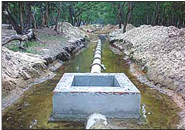
Fig.7 Construction of 11.23 Km Sewerage line for Digha
