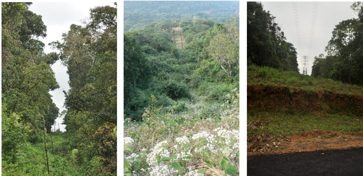
A transmission powerline fragmenting rainforest in Vazhachal, Kerala; weeds spreading along powerline clearing; double trouble of road and powerline each cutting its own swath through the forest (Photos: NCF)
