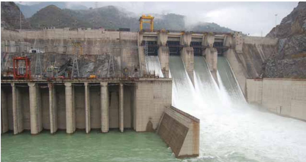
Photo 6.5: Koteswar Dam & Spillway
