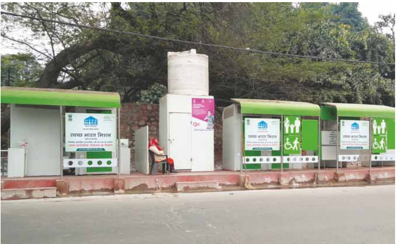
Photo 8.1: Toilets built under Swachh Bharat Mission
