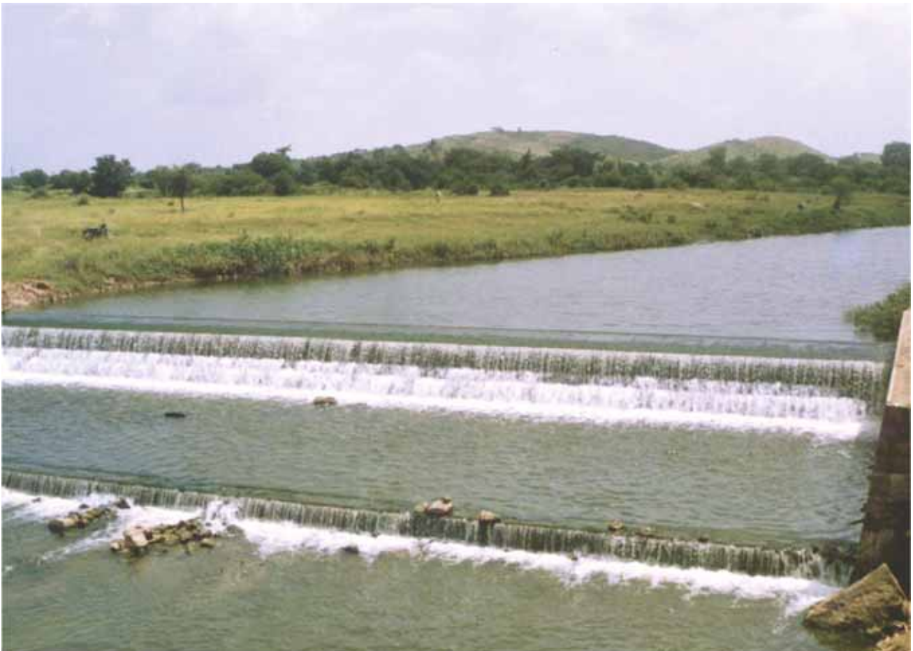
Photo 4.3: Check dam for water conservation in Bundelkhand
