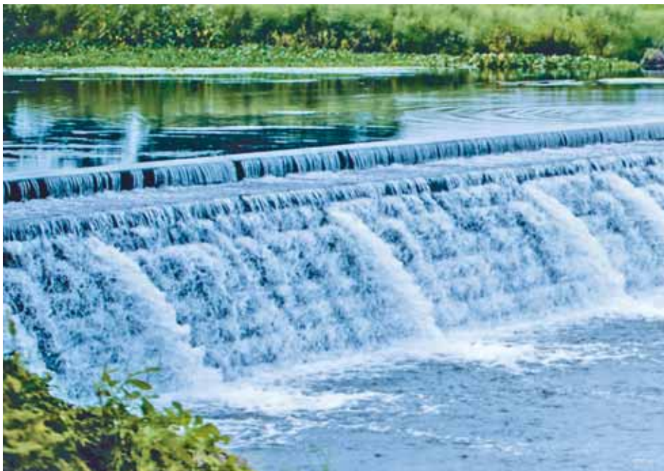
Photo 5.3: Construction of small dams under watershed management
