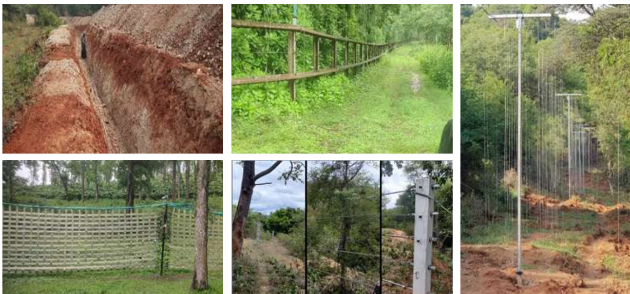
Fig-32: Types of Physical Barriers-Traditional EPT; Modern Fences- Railway Girder (KAR); Hanging Power Fence (All States); Steel Rope Fence (TN); AI-Smart Fence (KER)
